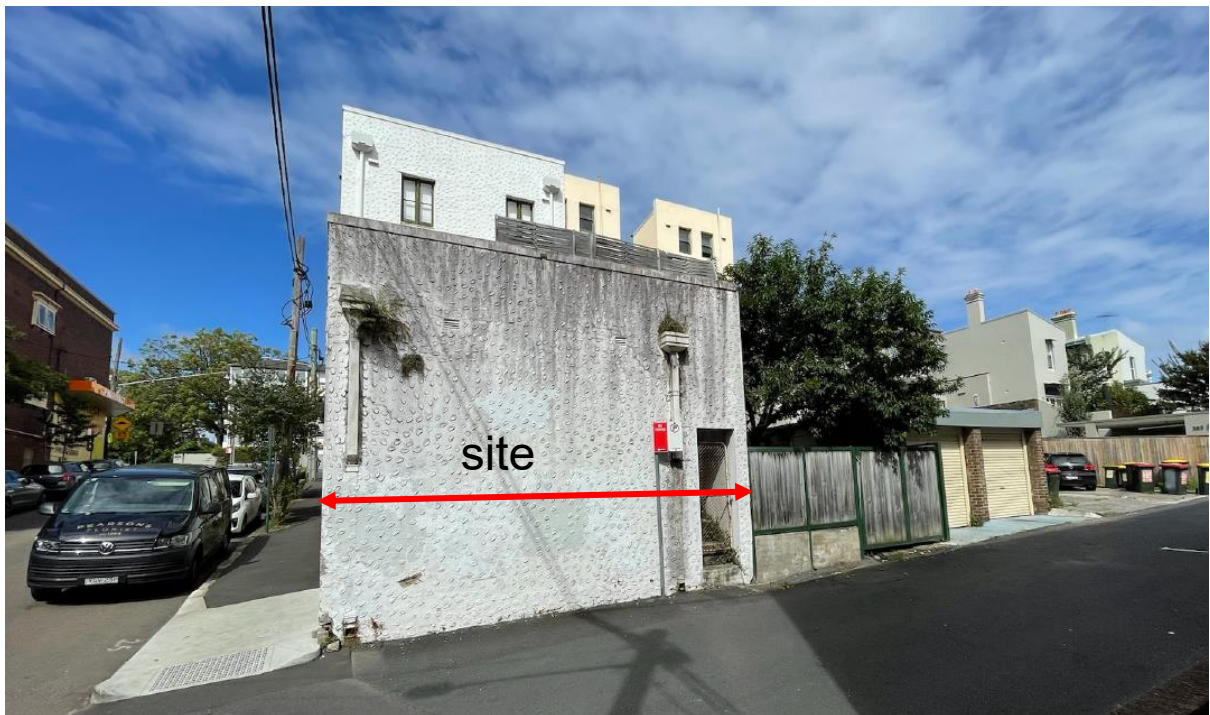
Figure 4: Rear of site and laneway viewed from Charlton Way
